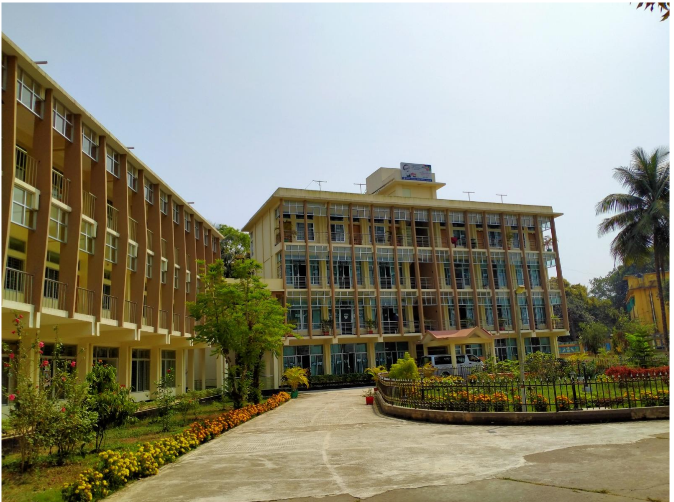
Academy Building of Engineering Academy, BPDB, Kaptai, Rangamati
